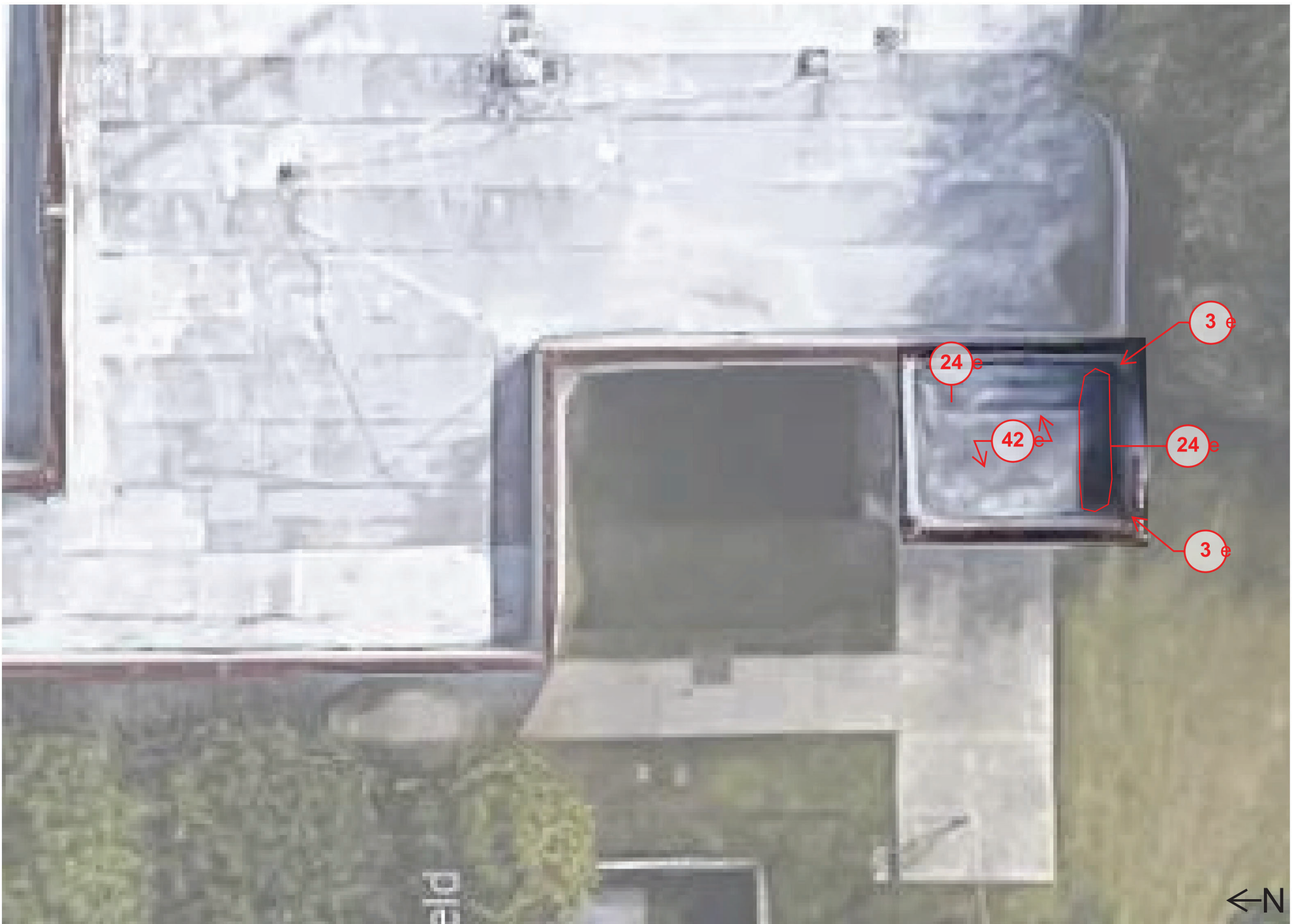
Building 0449 - West Airfield Station (ARFF) e Sector C e
